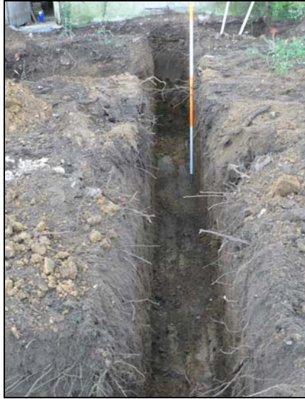
Main extension- western foundation trench from north
