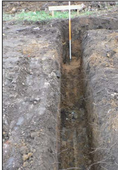
Main extension- central foundation trench from east
