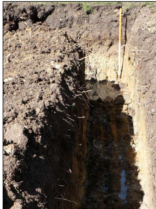
North-western corner of foundations
