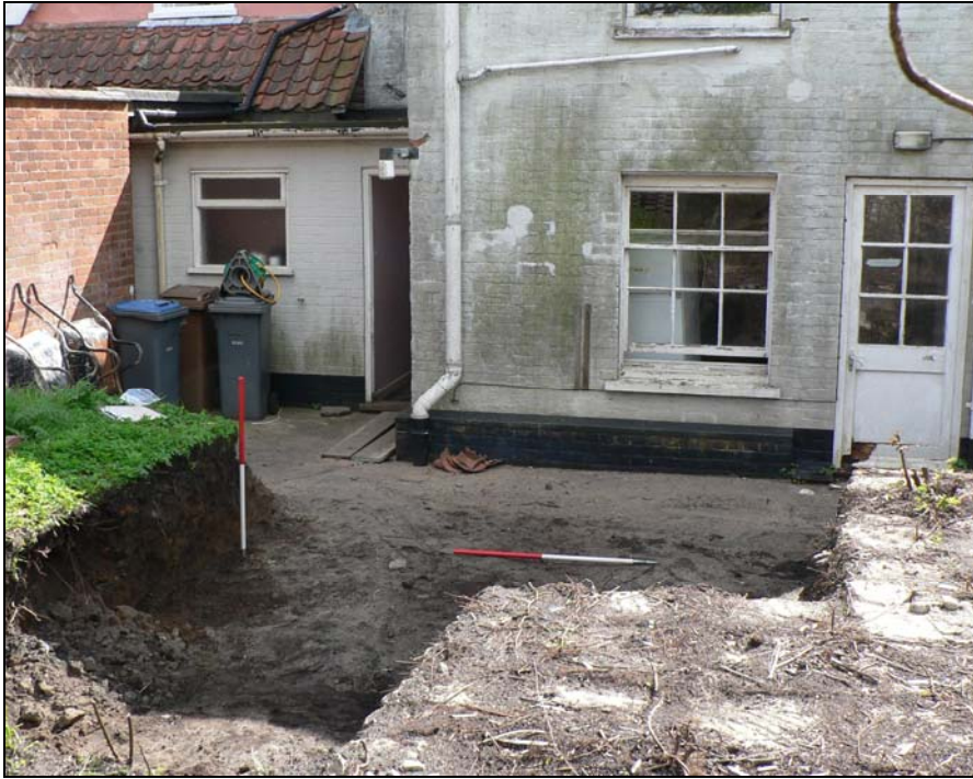
Phase 1 monitoring from west
