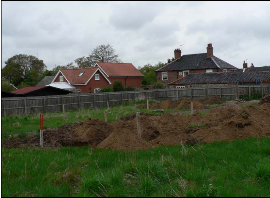
General view of site from south-west with the church & The Lion PH in background
