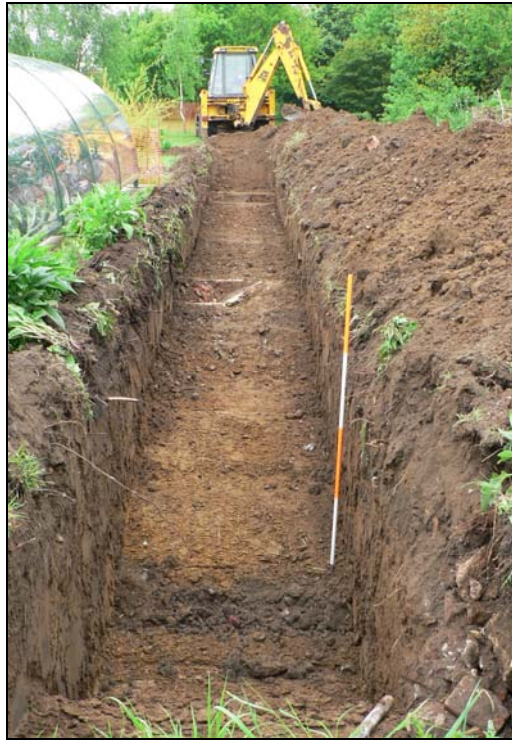
Trench from south
