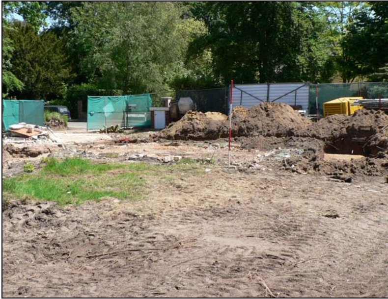
General view from south-west looking towards Gaston Street
