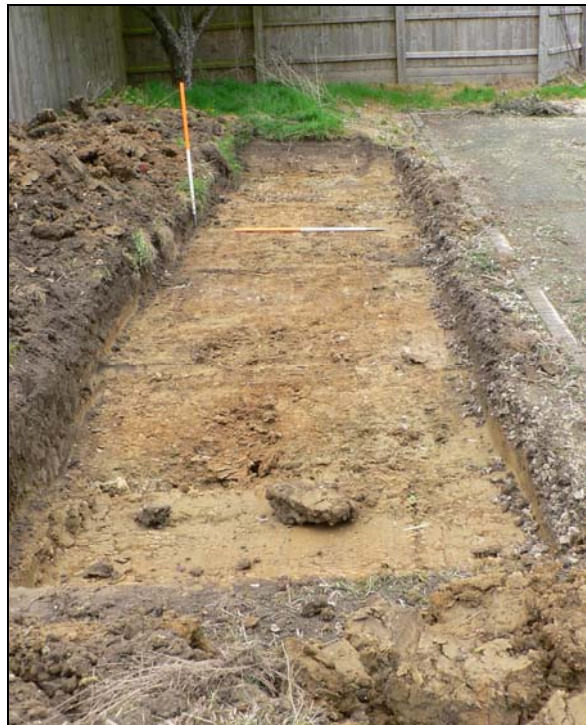
Trench 1 from west
