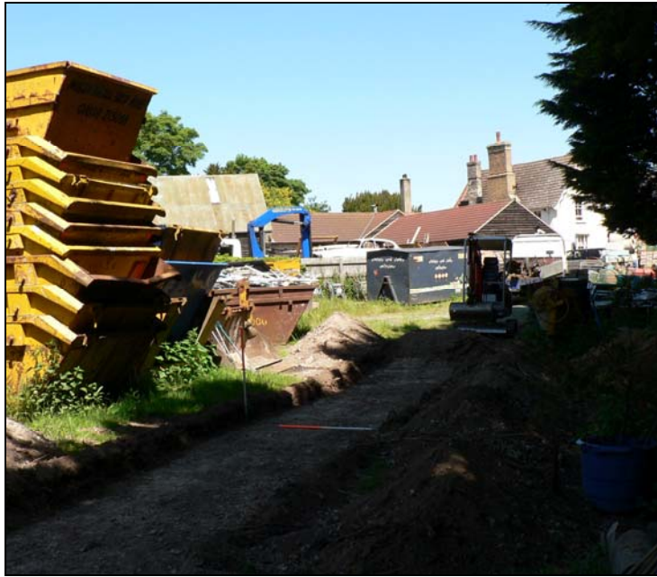
General view of site from south with farmhouse in background
