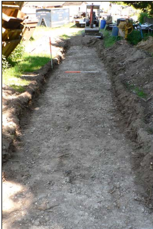
Trench from south
