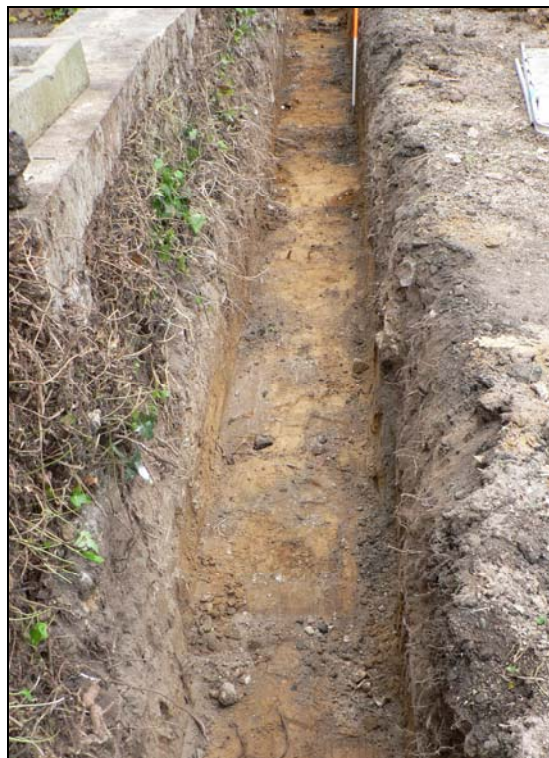
Southern foundation trench from east
