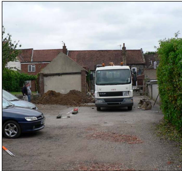
General view from east looking towards The Bell Inn
