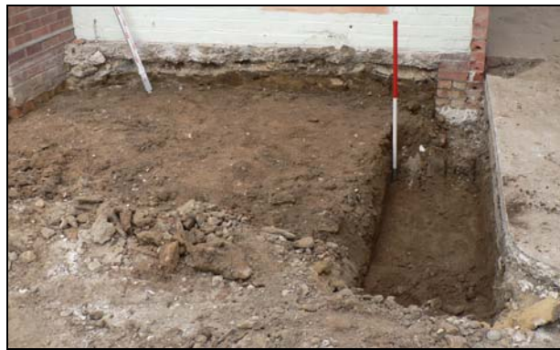
Rear extension raft excavation & toe round edge within subsoil
