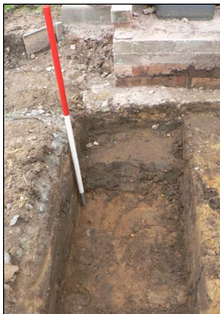
Front extension footing max depth to top of natural sand
