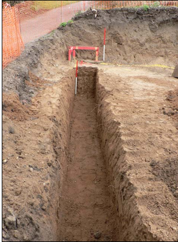
Western garage footing from south
