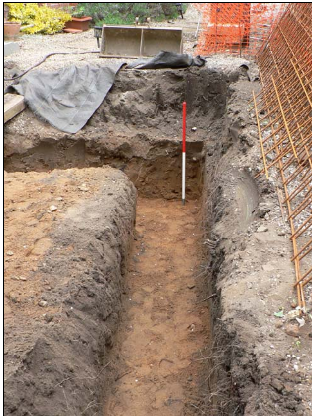
Orangery extension footing from west
