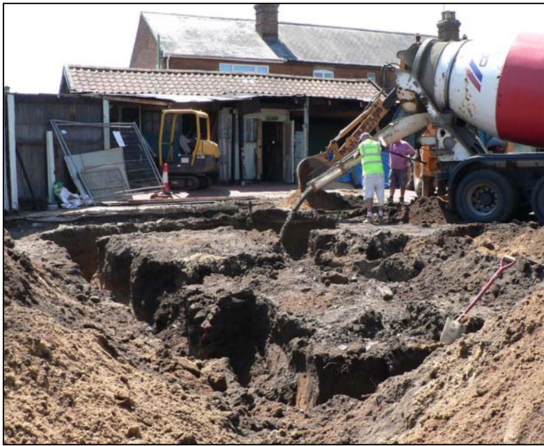
General view from north-east
