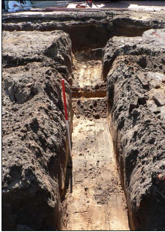
Typical foundation trench
