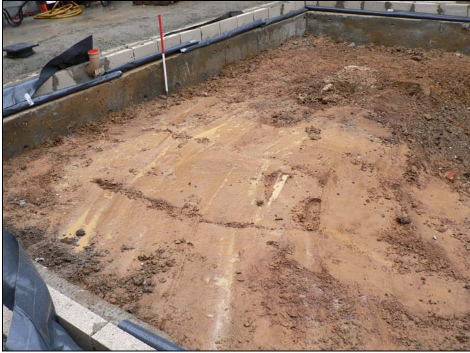
Monitoring following installation of ring beam
