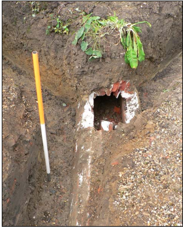
Brick culvert in service trench
