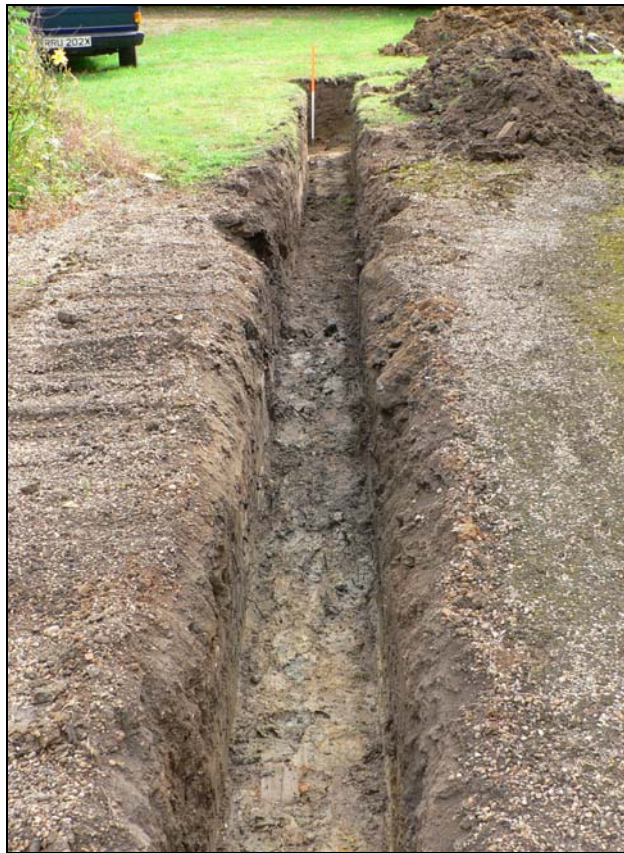
Service trench from west
