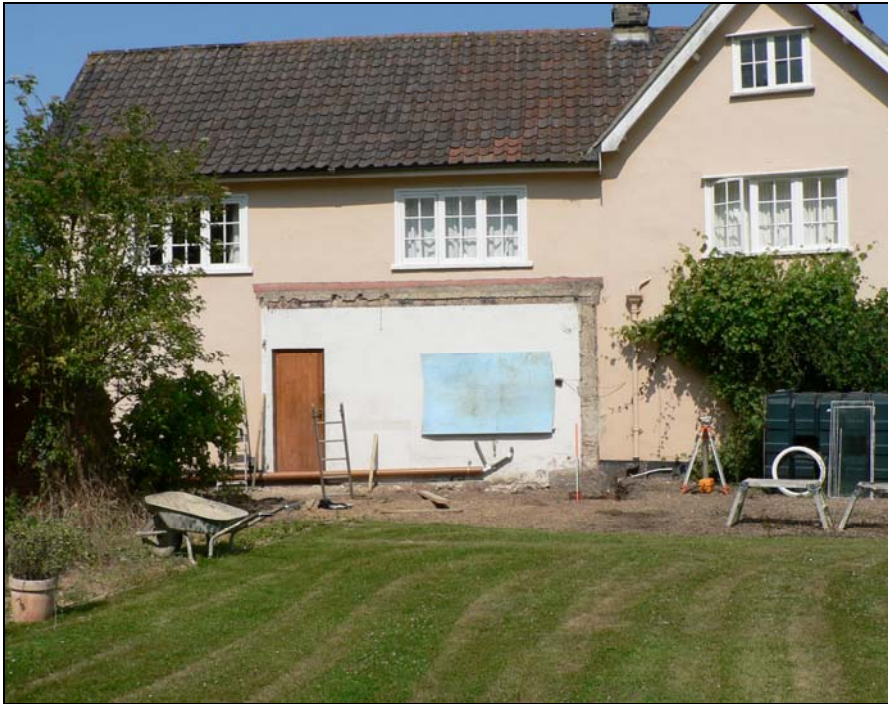
General view from west of extension area
