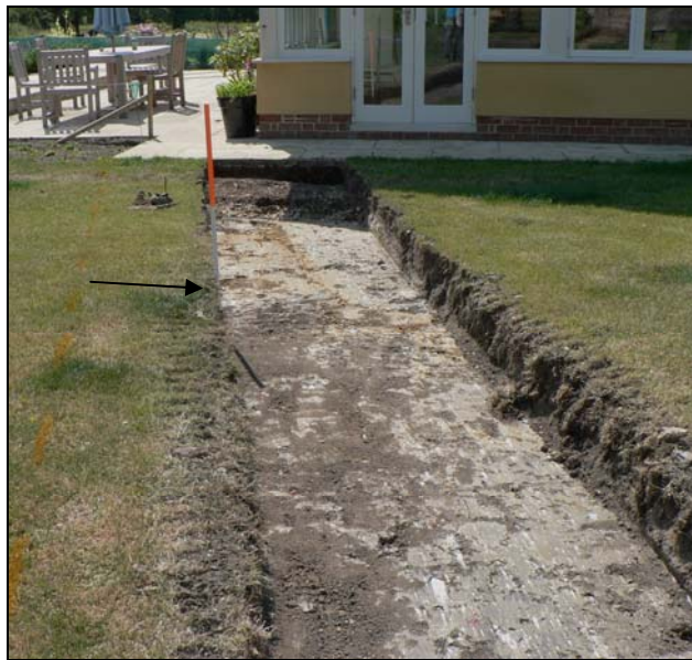
Soil strip from north-west with probable moat edge at mid-point (arrowed)
