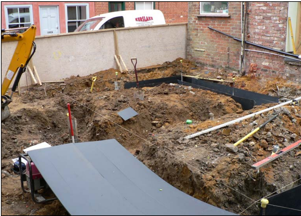
General view from south-west
