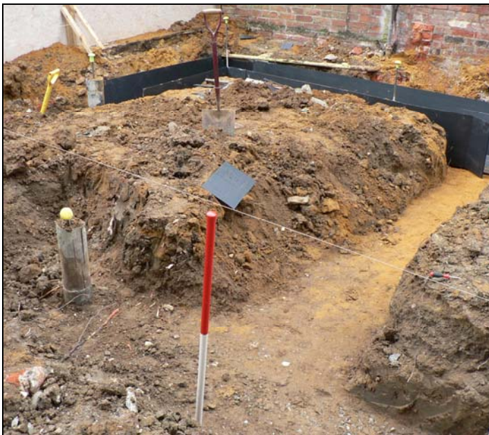
Ground beam trenches from west
