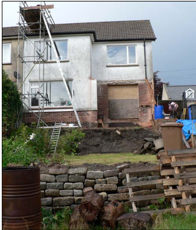
House from rear garden
