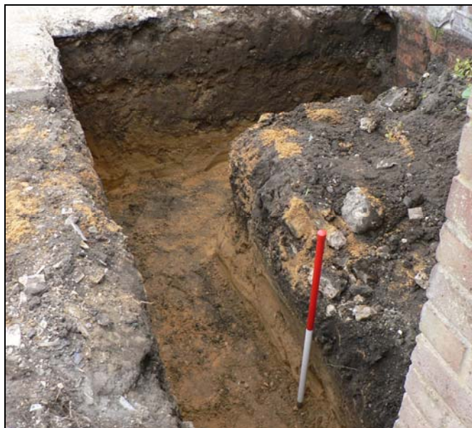
Foundation trench for front extension
