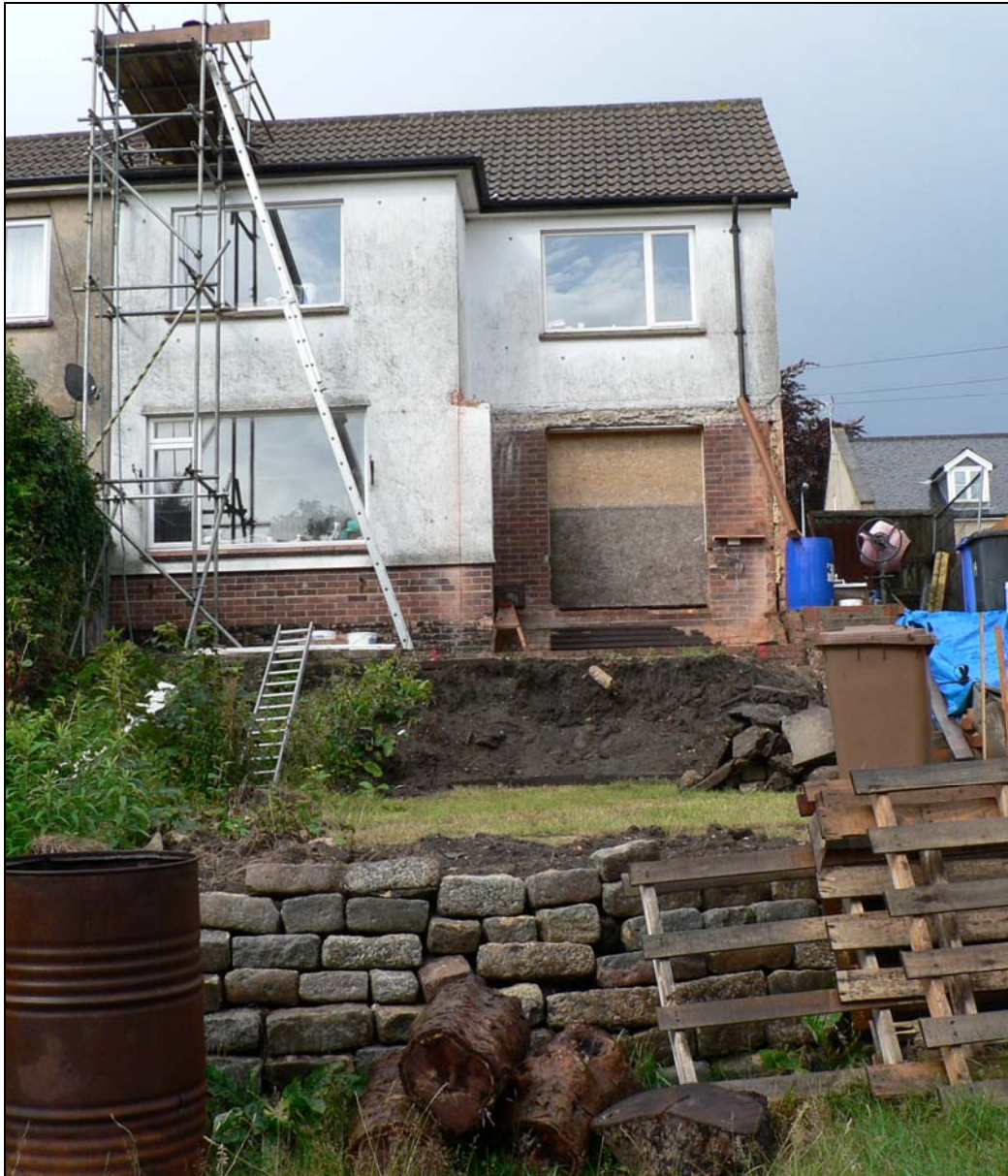
House from rear garden
