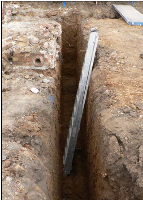
Foundation trench in middle of rear extensions from south
