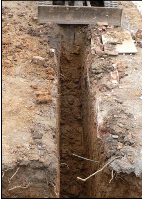
Trench for rear extension
