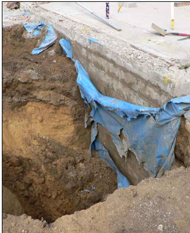
Late 20 th C cellar foundation disturbance to rear of hall
