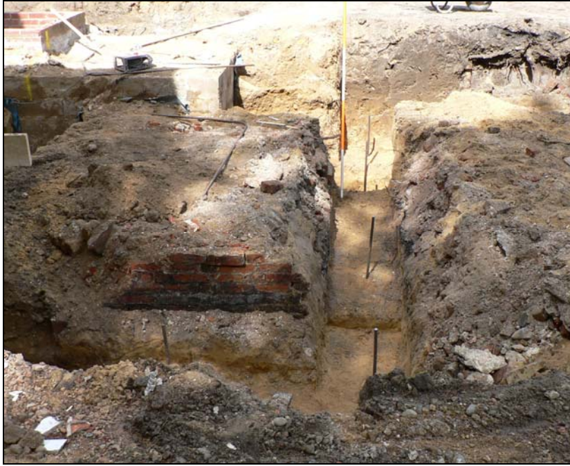
Side extension- remnant of mid 19 th C foundation
