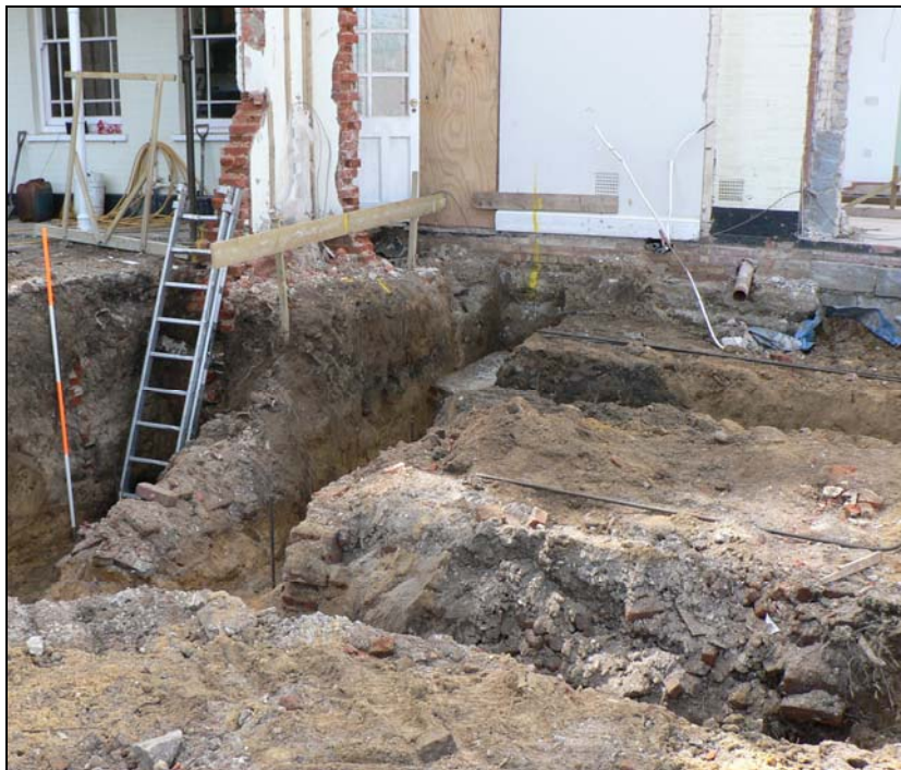
Side extension foundations from NW with probable infilled cellar entrance to right of scale pole
