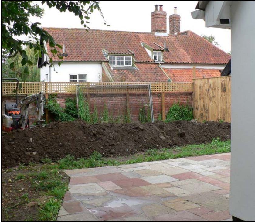
General view from south-west & yard of new dwelling
