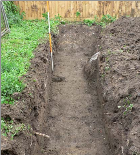
Trench from west (depth 1000mm)
