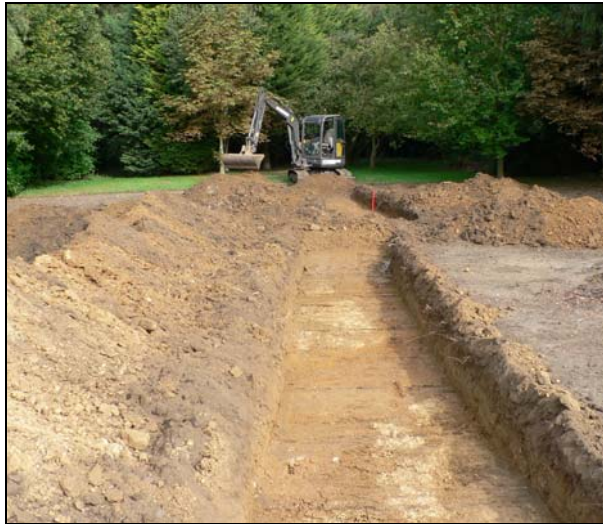
Trench 2 from west
