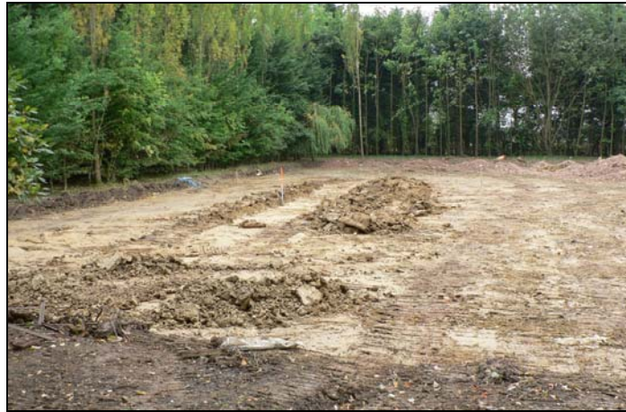
General view of stripped western area with T2 open
