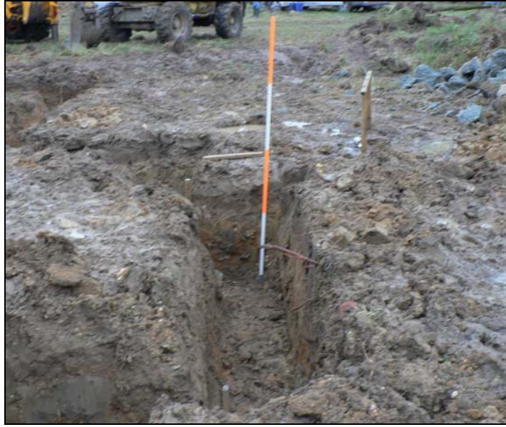
North-eastern corner of foundations
