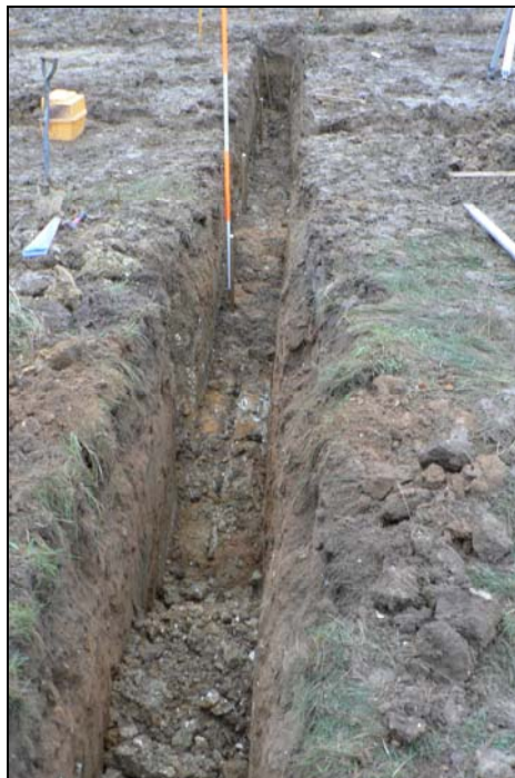
Western foundation trench from south
