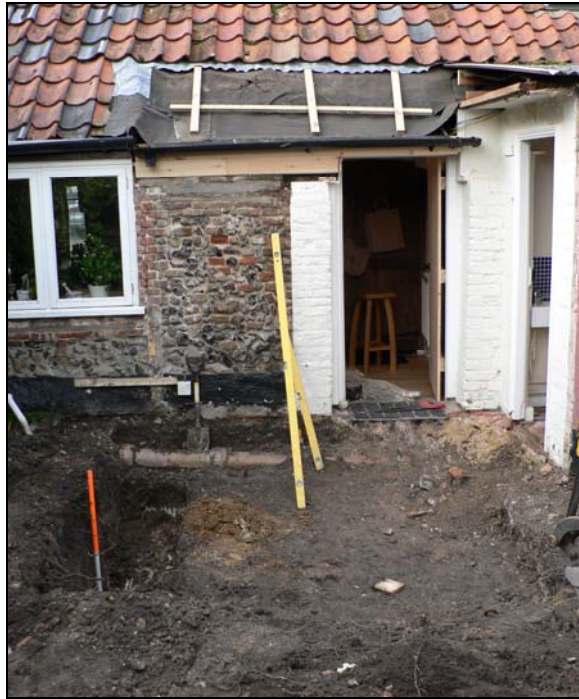
General view of the area of the rear extension
