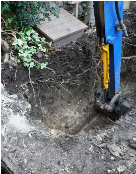
Eastern foundation trench from north
