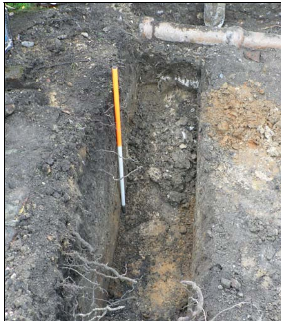
Western foundation trench from south
