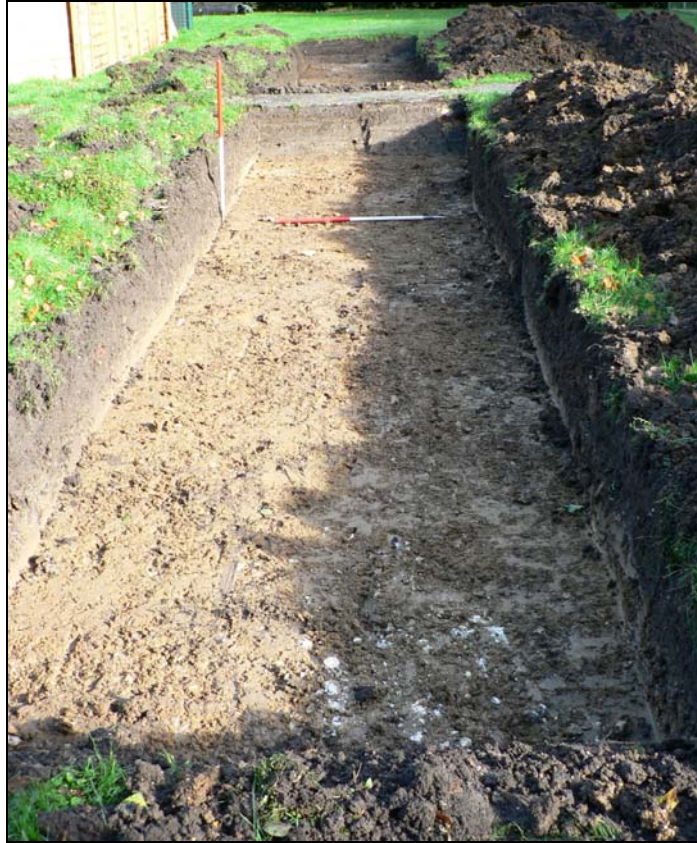
Trench from south-west
