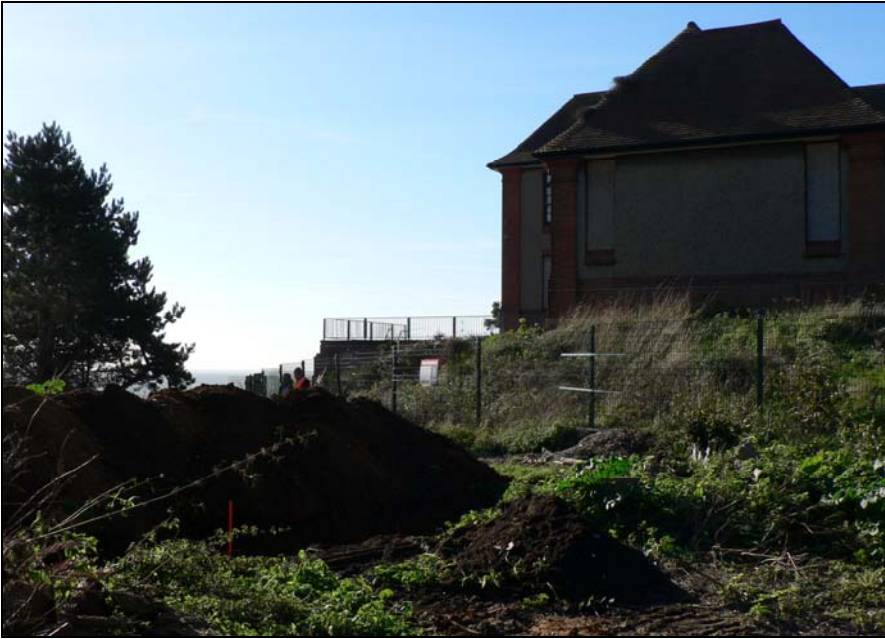
General view of eastern end of The Bartlett- trench 1 in foreground
