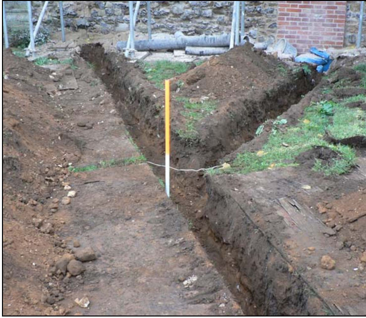
Trenching works on eastern side from east
