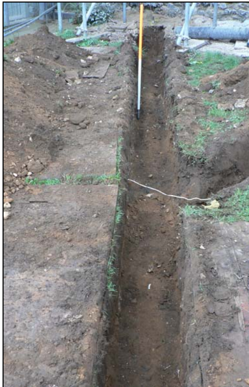
Pipe trench on eastern side from east
