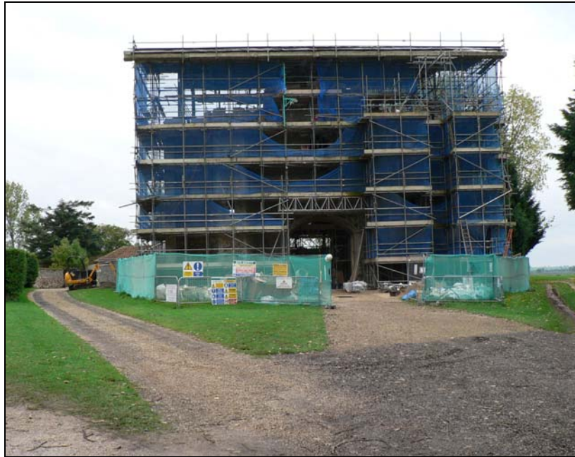
Pentney Abbey gatehouse during restoration from north
