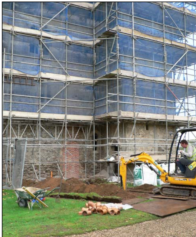
Area of trenching works on eastern side of the gatehouse
