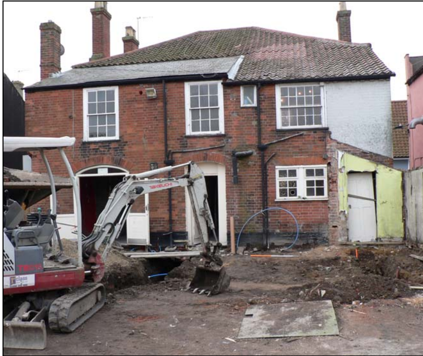
General view of rear of building from the north
