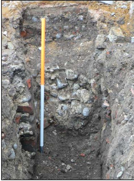
Flint & mortar under rear wall of building in western trench from the north
