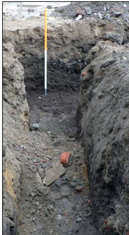
Western foundation trench from south
