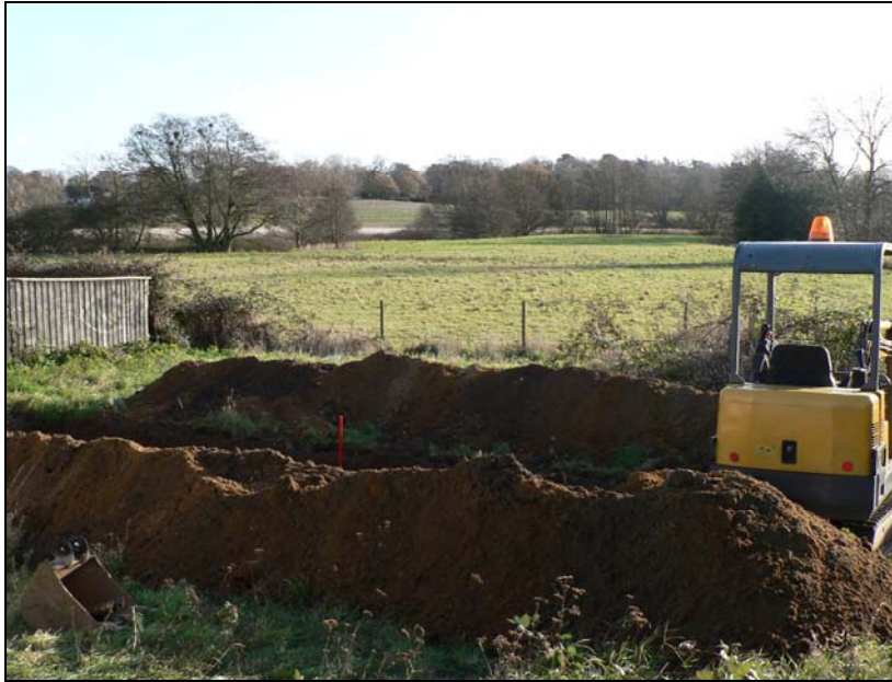
General view from northwest looking towards River Alde in background
