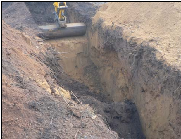
Trench 1 removal of topsoil for next length
