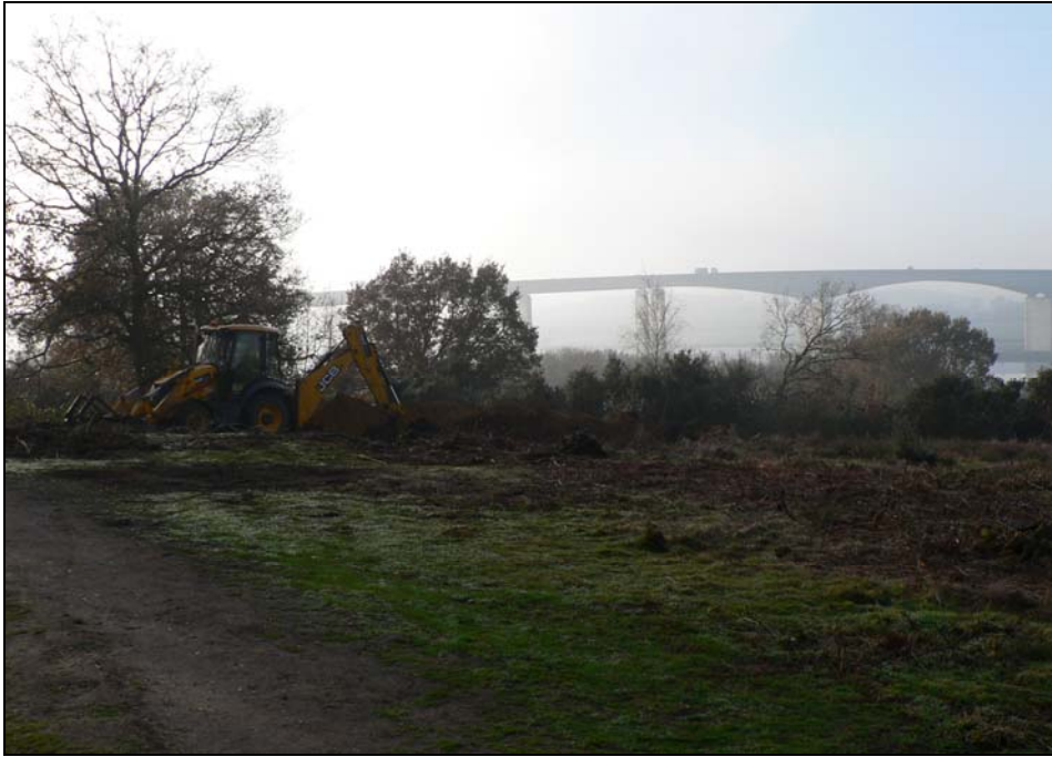
General view from north-west
