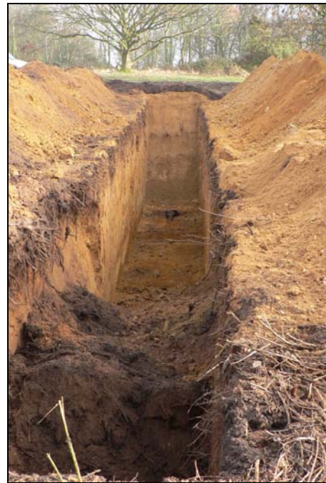
Trench 1 fully excavated
