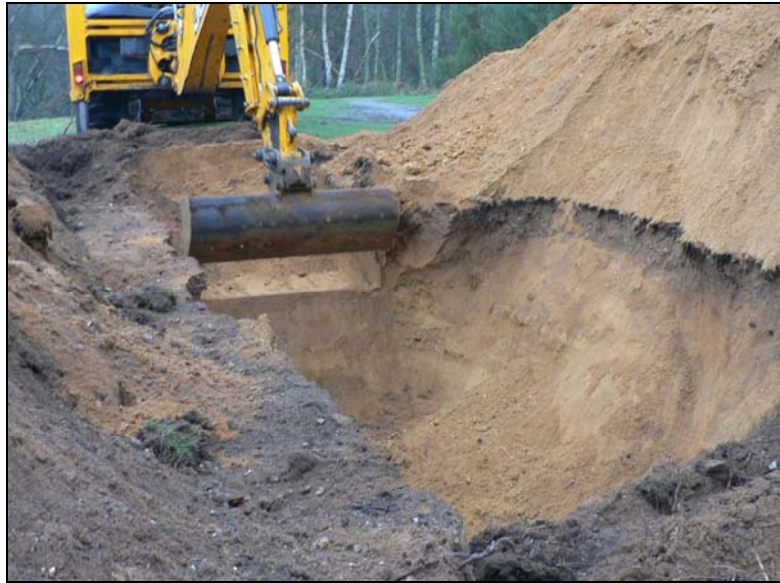
Trench deposit profile & removal of topsoil for next length
