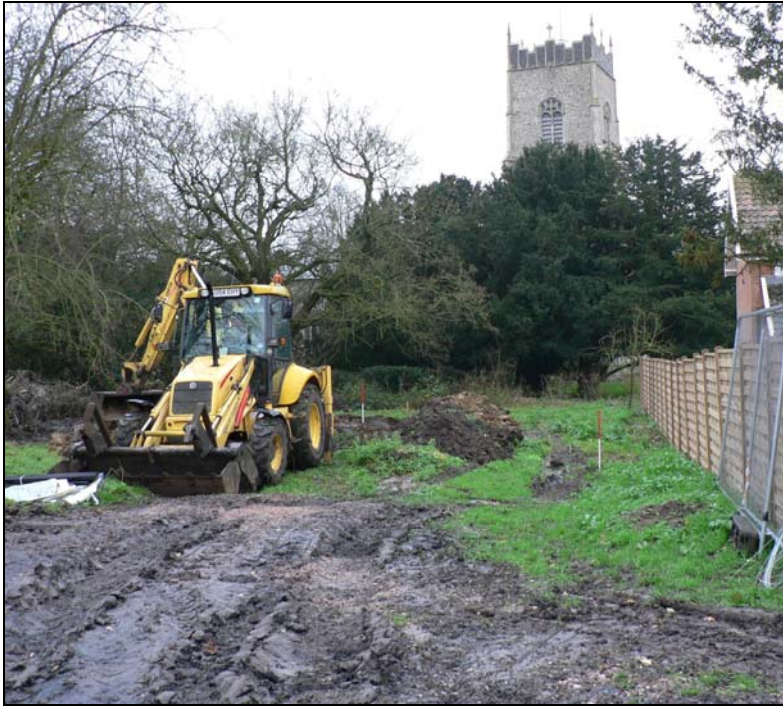
General view from north
