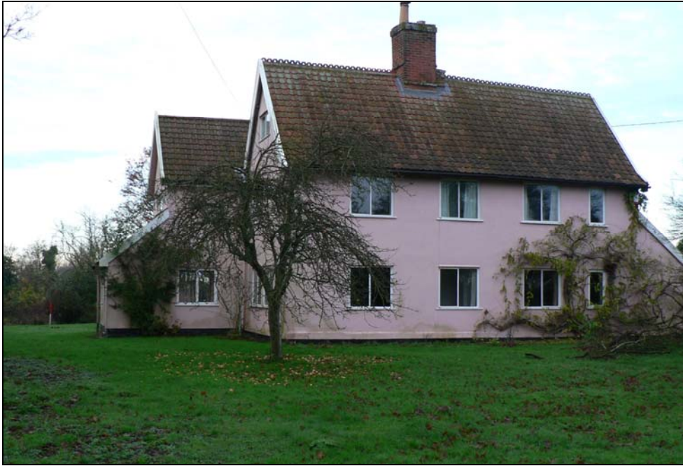
Church Farm House from east
