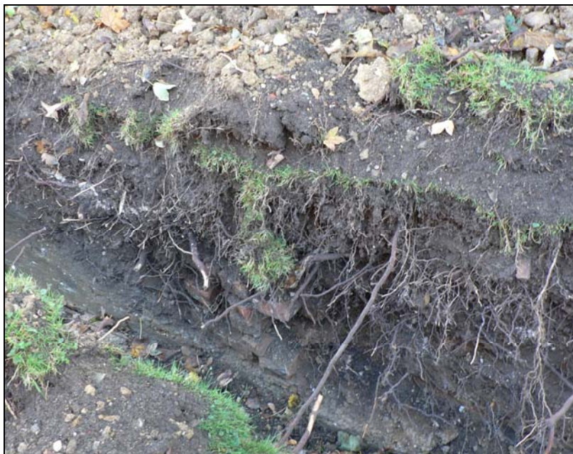
Brick soakaway in service trench
