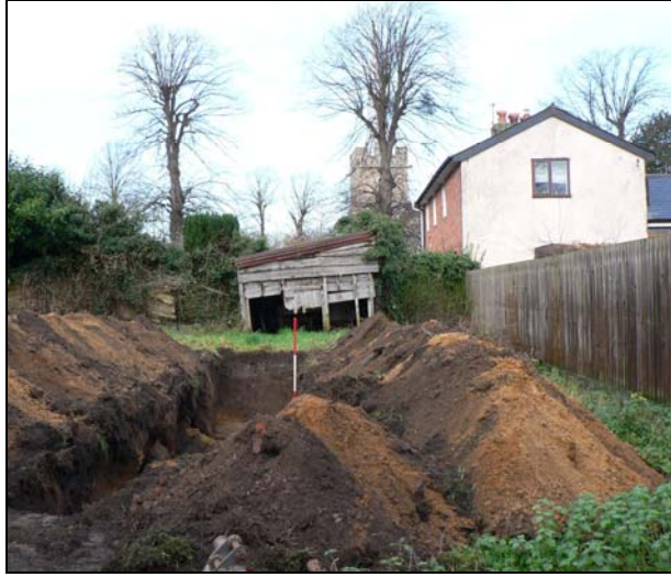
General view from east with church in background
