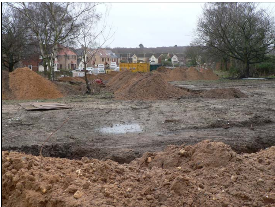
General view across north-eastern part of site from west
