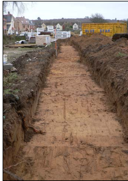
Trench 4 from west
