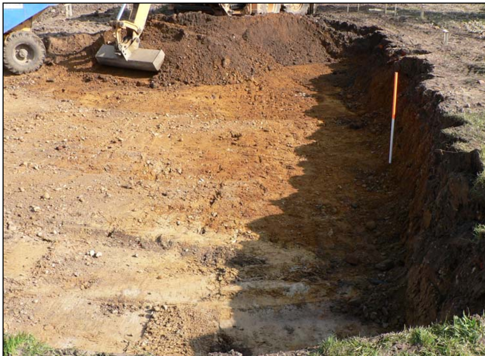
Ground reduction for garage/utility building
