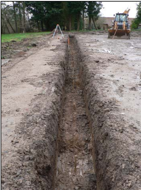
Eastern house footing from north
