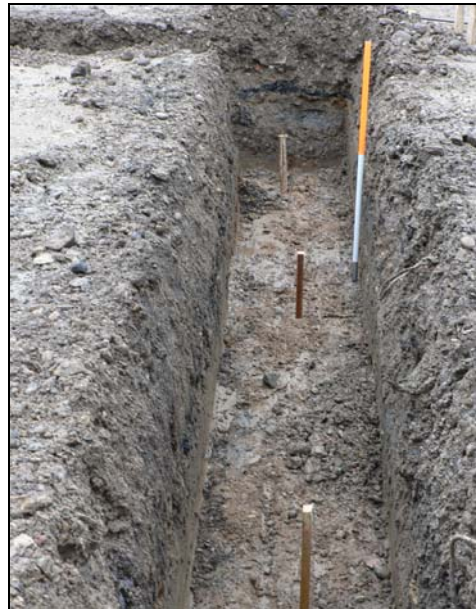
Western house footing from north
