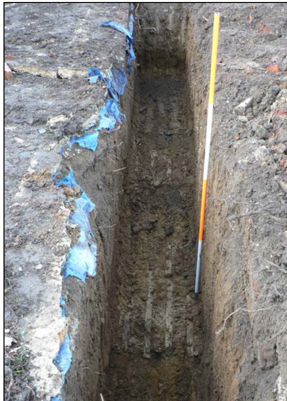
Southern foundation trench from east
