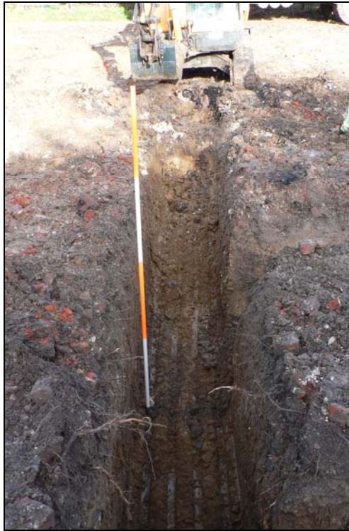
Eastern foundation trench from south
