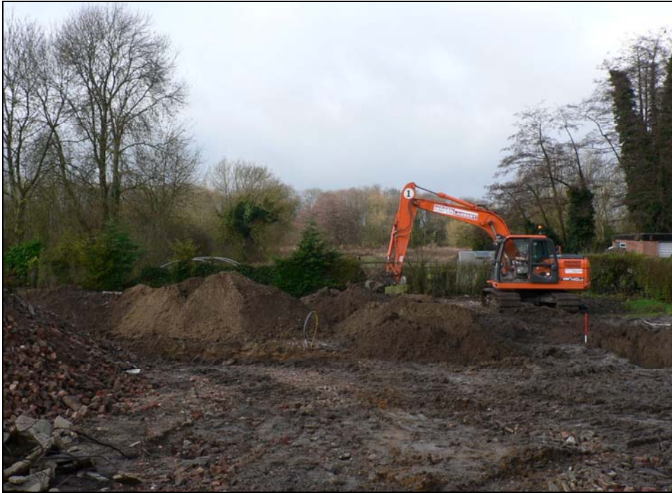
General view from east looking towards Black Bourn floodplain
