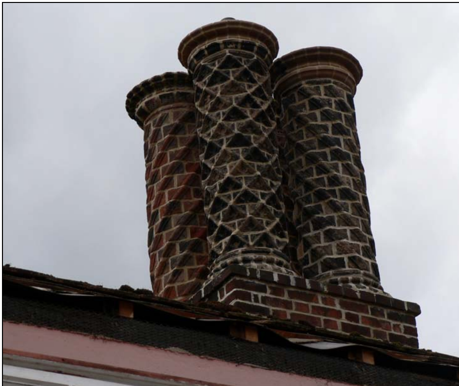
Detail of chimneys
