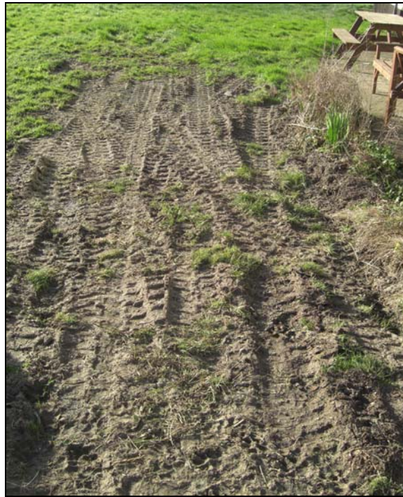
Area of trench 2 after back-filling
