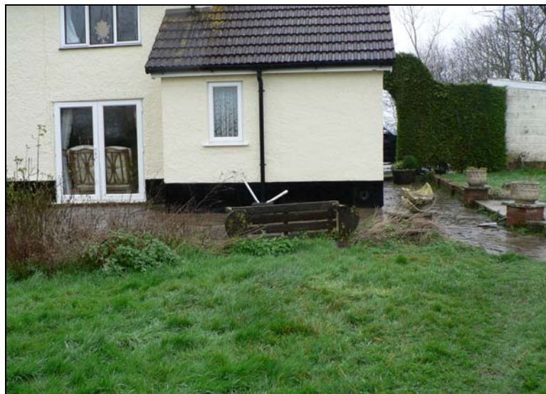
Area of trench 2 before trenching
