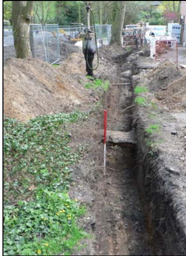
Pipe trench to north of Garden Lodge/Coach House from north-west
