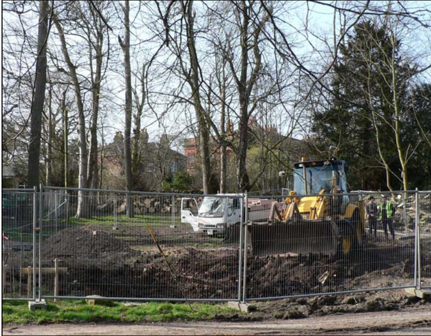
General view across boiler toward Redisham Hall from east
