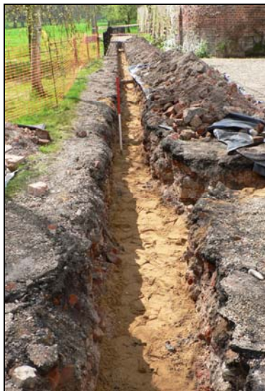
Cable trench to the east of the Coach House from north
