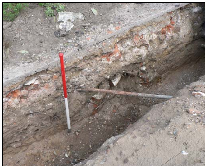
Brick built well/soakaway to south-east of West Lodge
