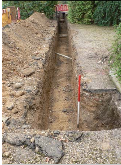
Pipe trench in front of hall from north-west
