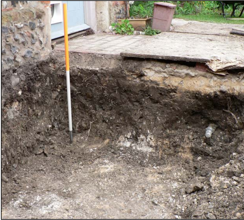
North-eastern corner of raft foundation
