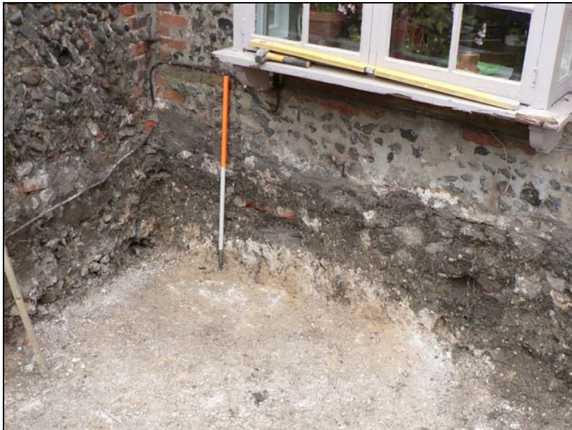
North-western corner of raft foundation
