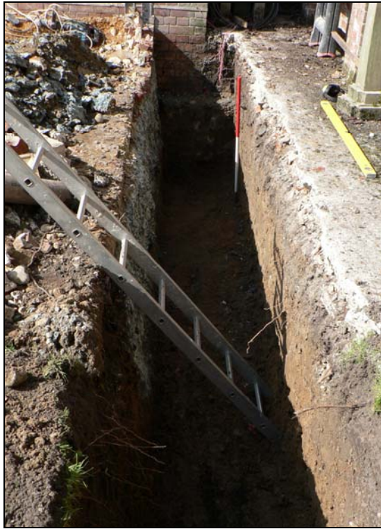
North-western length of extension trench
