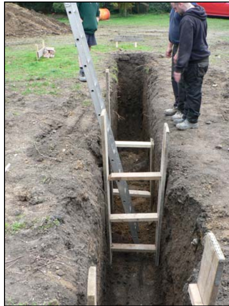
Eastern trench from north
