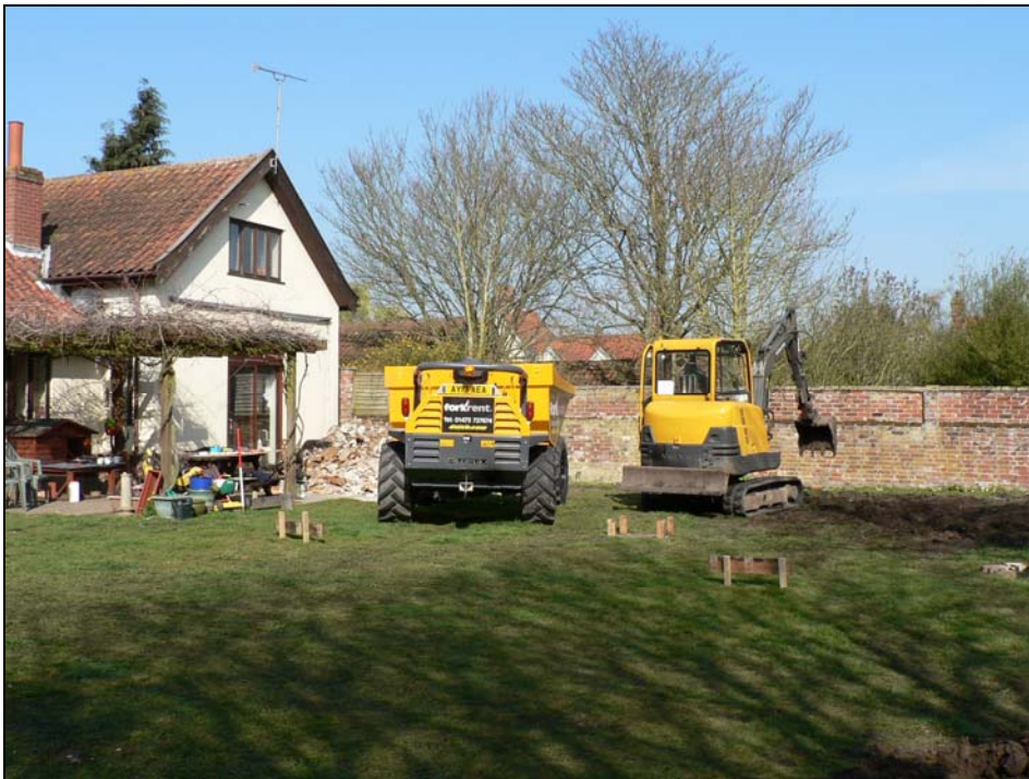
General view of extension area from south-east
