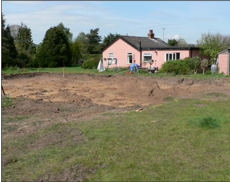
General view from southeast
