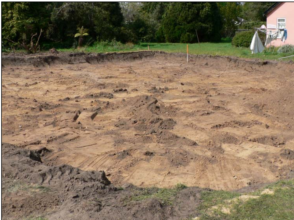
Stripped area from southeast
