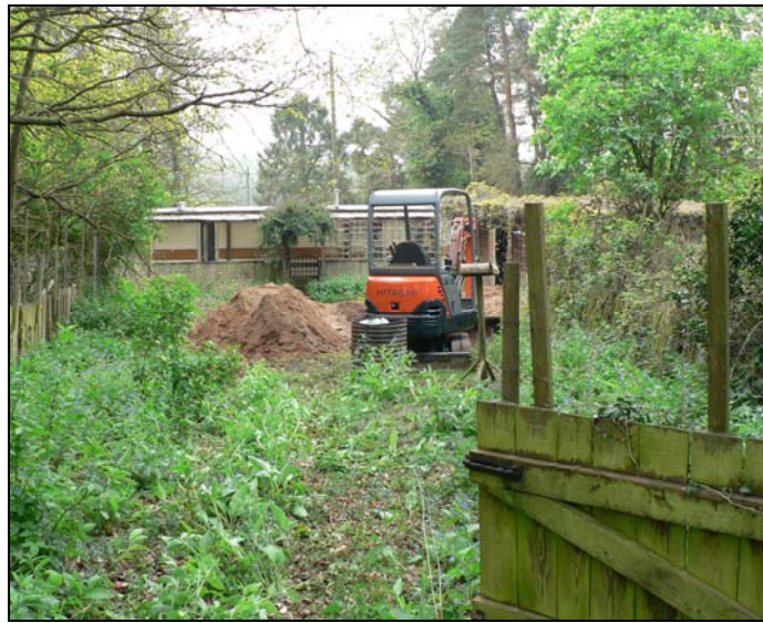
General view from north
