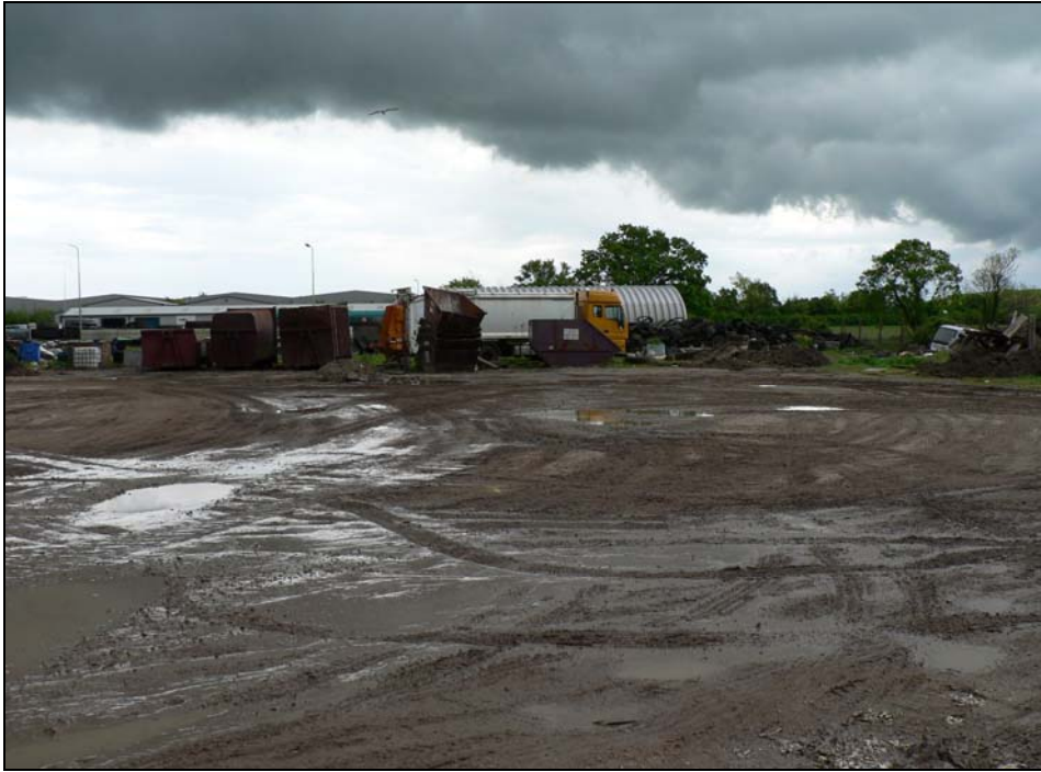
General view from west
