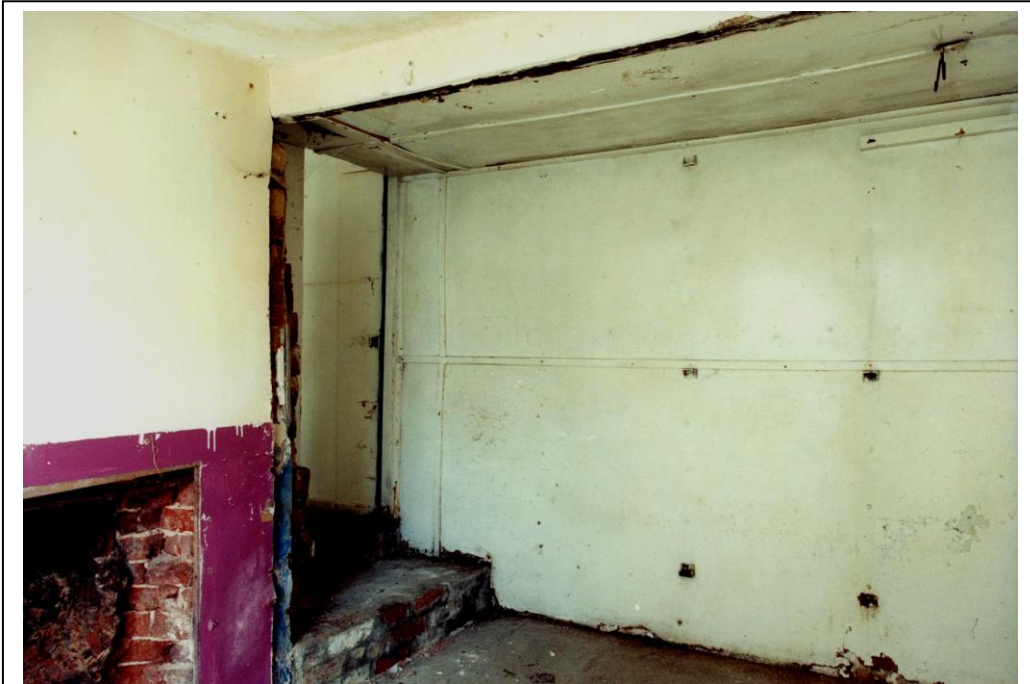
Fig. 19: Rooms G2 and G3, looking north-west
