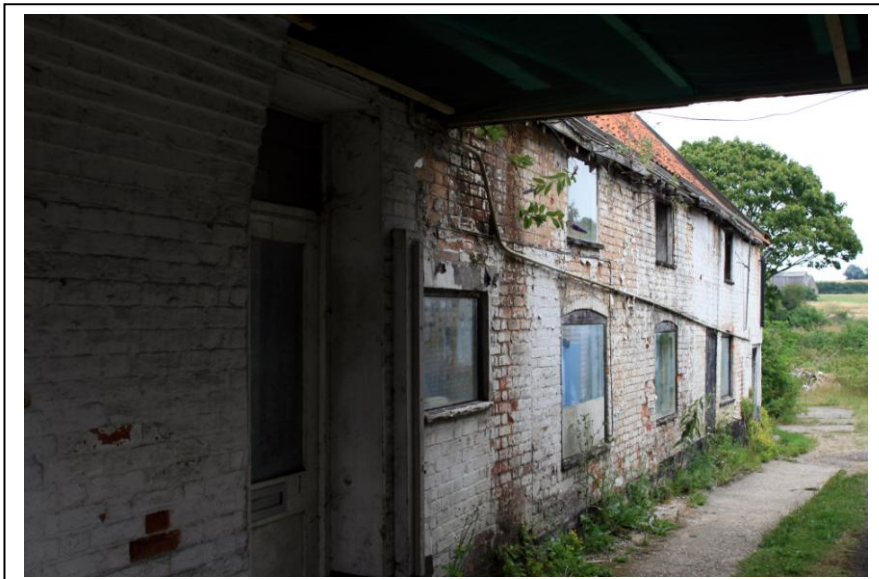
Fig. 2: South elevation towards the yard, looking east
