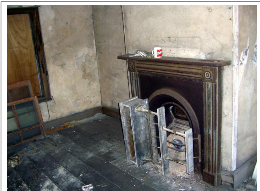
Fig. 13: Room F1, over the carriageway, north and west walls
