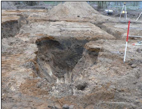
Plot 9 central area of foundation trenches
