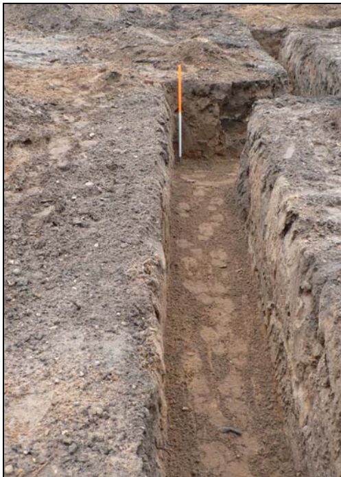
Plot 10 eastern foundation from north
