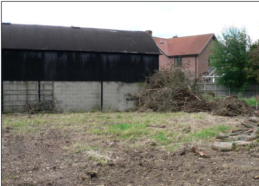
General view from north
