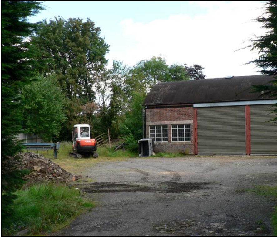
General view from south (road edge)
