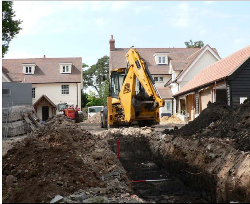
General view from north
