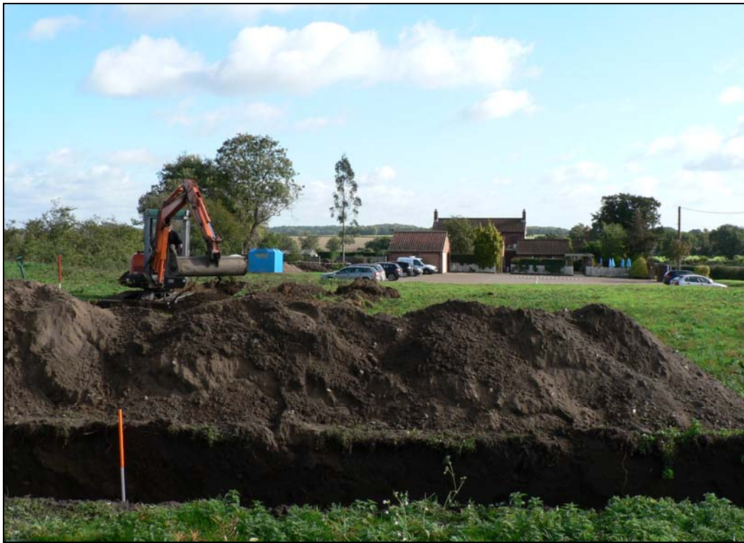
General view from west
